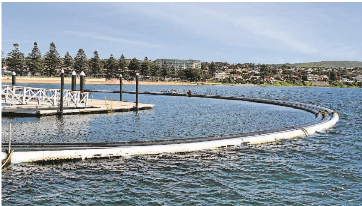
Figure 3: Attenuation of small waves by the floating tubes.
