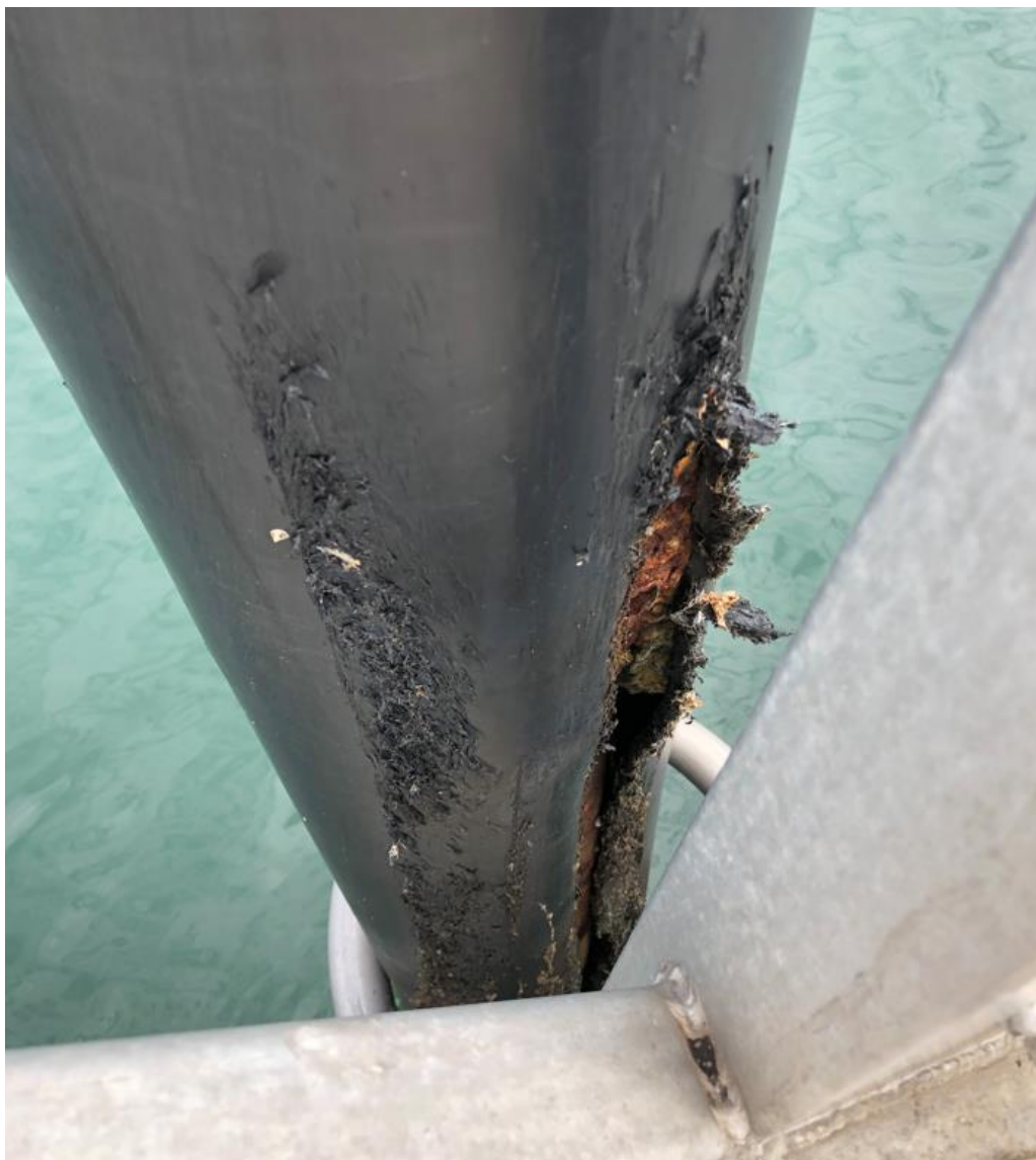
Figure 2: Photograph taken on 13 September 2022 showing the penetration of the HDPE sleeve to the pile at pontoon unit P10.
